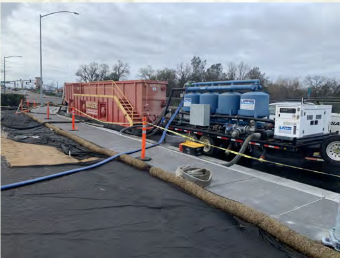
ATS will customize the treatment system to fit your stormwater needs; Pictured: 300 GPM Mobile ATS
